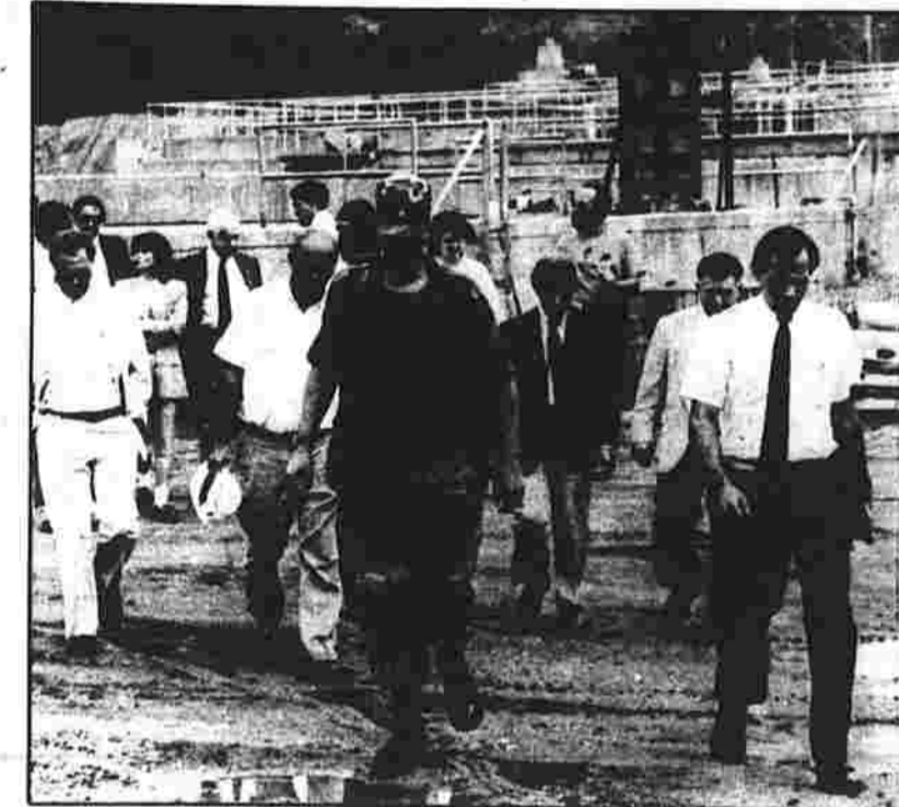
TOURING PLANT — Lt. Col. Stanley J. Murphy, deputy division engineer for the New England division of the Army Corps of Engineers, and Robert J. Young, superintendent of the town's Water and Sewer Division, lead a July 12 tour of the construction site for an addition to the town's sewage treatment plant.
